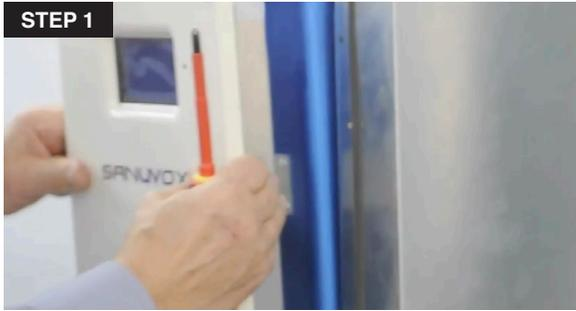
1. Take the R Max out from the ductwork by removing the 4 screws located on the cover (4 corners) that hold it to the frame.
