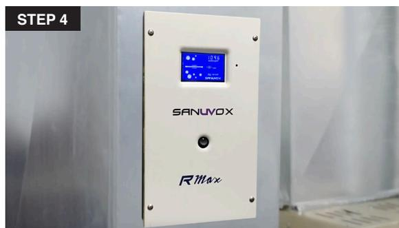
4. From now on, the R Max will only activate the lamp when the thermistor detects airflow in your duct system.
