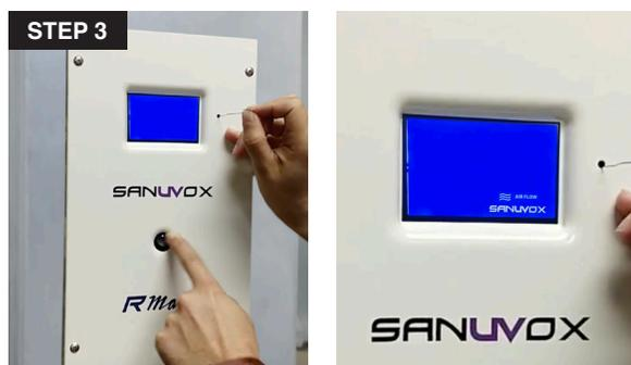
3. First turn ON the power switch and then, press the reset button. You have 5 seconds from the moment the unit is powered to press the reset button to activate the airflow detection. Every time you press the button you will notice the word "AIR" appears or disappears from the bottom right corner of the LCD screen. Once "AIR" appears on the screen, wait for the lamp to turn on so that the setting is saved.
