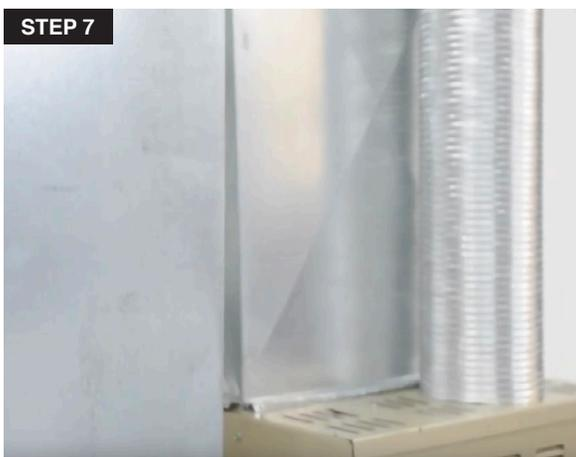
7. Prepare the duct (return or supply) for installation. Evaluate the ideal area for installing the air purifier. **The reflection chamber should always be parallel to the airflow.** Ensure that the purifier will fit into the plenum and position it keeping in mind to minimize plastic exposure to direct UV light.
