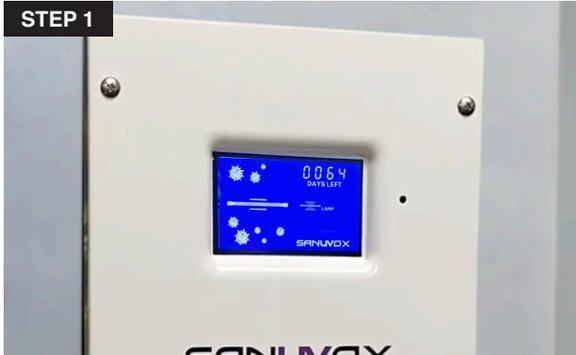
1. To reset the lamp timer the unit needs to be powered and turned ON. The LCD status should be on 'Stand-by' or 'Active'.
